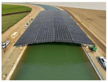
This project is designed as a "proof of concept" to determine if this type of installation could be used on the many miles of water canals in California (most of which are agricultural canals used for irrigation of crops).
