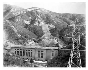
A 1928 view of an early Los Angeles Aqueduct hydroelectric facility, showing the powerhouse in the canyon, the 115 kV transmission tower in the foreground, and the steep penstocks carrying highpressure water down to the turbines. Completed in the 1910s, it was the first hydroelectric powerhouse built by the City of Los Angeles to deliver commercial electricity to its residents. Remarkably, this historic facility still operates today, more than a century after it first began generating power.
